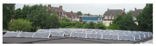
In May 2008 Ardenham Energy installed and commissioned the 6.68 flat roof mounted grid tied PV system on the gymnasium roof of the Claremont Primary School in Tunbridge Wells. The project was funded by the Kent County Council Renewable Energy Fund, Low Carbon Building Phase1 grant and from an Eon Source grant.
